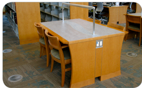
TAF-R diffusers with swirl face installed in the floor of a library
