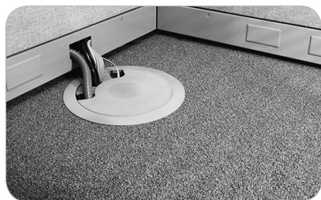
TAF-G diffuser installed in the floor of an office cubicle
